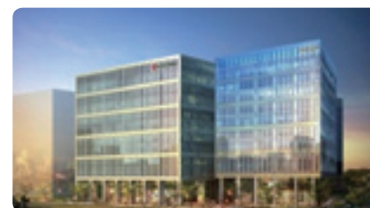
NAVER company building
